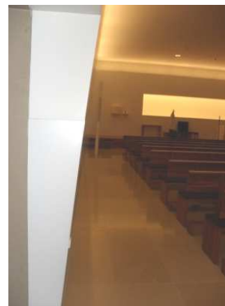
Figures 6 and 7 - Cushioned pews (top) and the slope of the wall panels to minimize multiple reflections (bottom).
