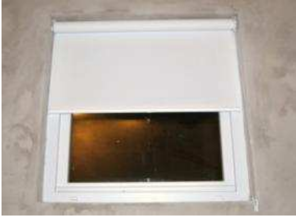
Fig. 8 and 9 – Application of the screens by the outside of the opening 8) exterior screen, half closed, on opening #1; 9) exterior screen on opening # 2, entirely closed.
