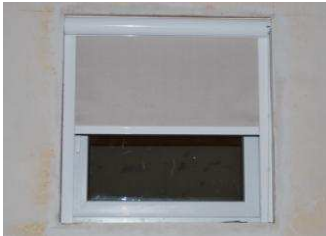
Fig. 10 and 11 - 10) Schematic cut of the window and interior screen; 11) Opening #1 with the opaque interior screen, half closed.
