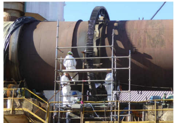
Figure 6 – Spring plates. a) Zoom of Figure 1, showing the toothed crown and spring plates (identified with arrows), undergoing repair/assembly work by technical staff.
