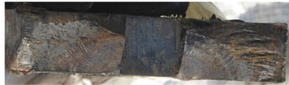
a) crack surface (represented by interrupted line AA in previous Figure 7).
