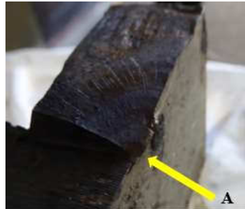
b) Detail of the crack propagation, starting at corner. Figure 8 – Crack surface of one of the broken eyebars.
