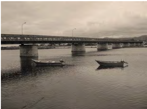
Figure 1 - Fão riveted road bridge
